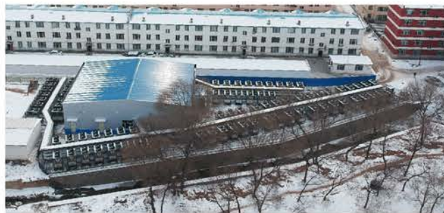
Helingeer Town, the Nei Monggol Autonomous Region Heating Area: 100,000m 2 Heat Pump: 150kW/unit Total: 80Units
