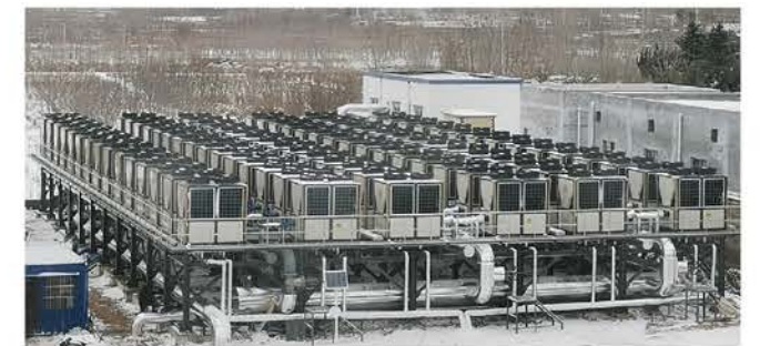
Cuipinglijing Community, Pingyin Meigui Town, Ji Nan City Heating Area: 300,000m 2 Heat Pump: 150kW/unit Total: 90Units
